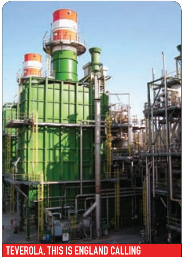
Photo courtesy of Emerson Process Management
