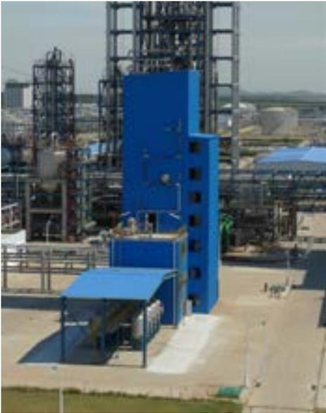
Chromium-based catalyst activator systems from Bigelow-Liptak are high-temperature, multi-zone systems used in the polymerization of High Density Polyethylene (HDPE). They are designed to satisfy the most stringent of petrochemical specifications, quality control standards and operational safety requirements.
